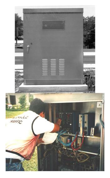
The field wires from the cabinet run through conduit that is encased in the cabinet foundation. Larger cabinets are typically ground mounted because of their considerable size and weight. Unless extenuating circumstances prevent it, the cabinet door should open away from the intersection. This allows the technician to easily monitor signal head indications and traffic behavior while, at the same time, observing the operation of the controller and detector units located within the cabinet.
