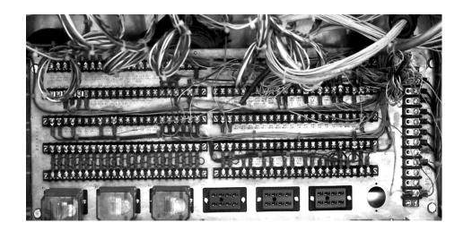
Decisions made by the controller are communicated, via the back panel, to the load switches which are plugged into the load switch bays on the back panel. The load switches then activate the field terminals which turn the signal heads red, yellow, and green. In addition, vehicle detections are input to the controller via the detector amplifiers which are also wired to the back panel.
