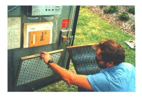
The cabinet cannot be completely sealed from water since air input vents are needed for the air circulation system to work. Consequently, if the cabinet is located close to the road and the door opens toward the road, passing vehicles may splash puddled water through the air input vents and into the cabinet. This is another reason to orient the cabinet so that the door opens away from the intersection.
