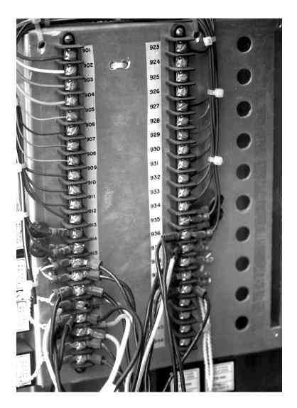
The field wires from the inductance loops are attached to terminals located on the detector panel. In many cabinets, field wires from the pedestrian detectors are also terminated on this panel.
